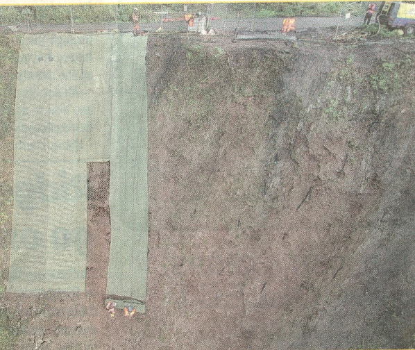
Matting being installed to stabilise the cliff face
