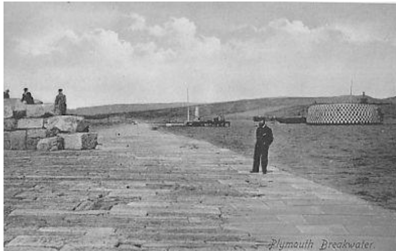
Workmen on the Plymouth Breakwater. Note the Breakwater Fort on the right. From a postcard.
