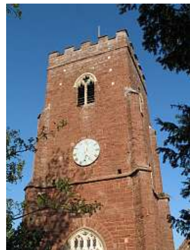
Exminster Church tower built in local Heavitree Breccia. © DJC Laming
