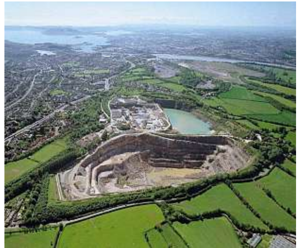
Moorcroft Quarry in Plymouth Limestone, east of Plymouth at Elburton. City Centre and Plymouth Sound far left. © Aggregate Industries
