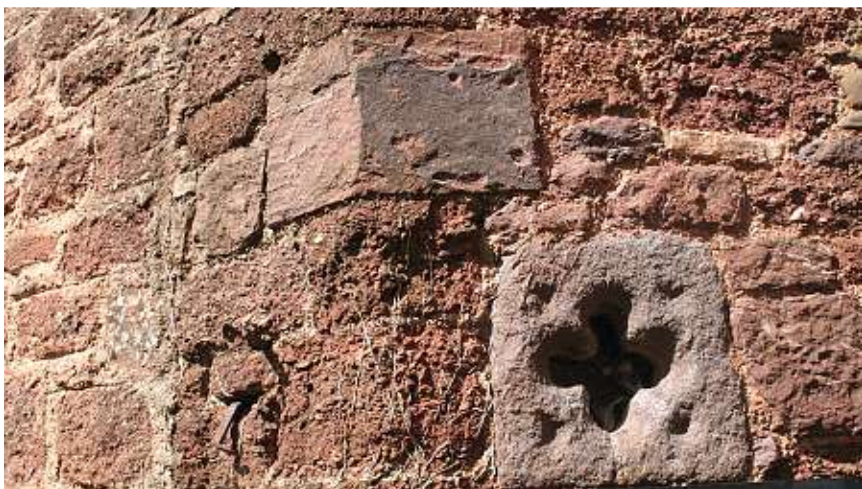
Exeter city building stones in local Permian red rocks – Heavitree Breccia, Pocombe Lava and Rougemont Basalt – at St Nicholas' Priory. © DJC Laming
