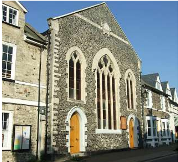
Ecclesiastical architecture using Beer stone for door and window details with flint for main walls. Congregational Church, Fore St, Beer. ©DW Allen
