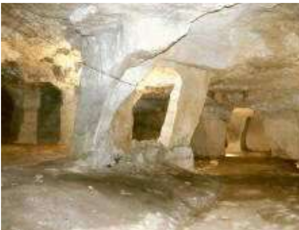
Underground quarry workings in Beer Stone, at Beer Quarry Caves - between Branscombe and Beer. © Beer Caves
