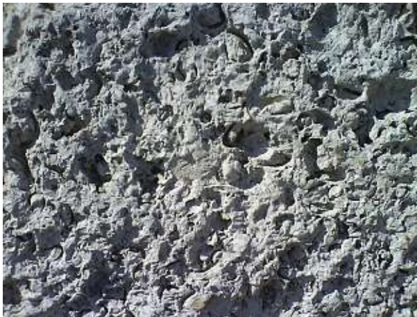
Jurassic limestone building stone full of shelly fossil debris in Lyme Regis. © DP Roche
