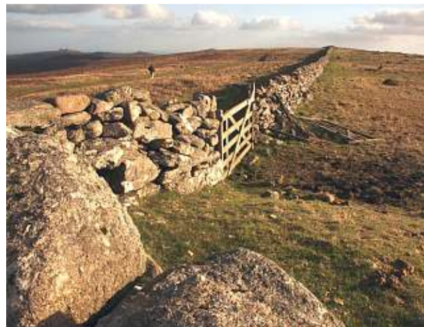
A high moorland Dartmoor Granite dry-stone wall, at Hameldown, near Widcombe. Photo DG5. © Clive Nicholas
