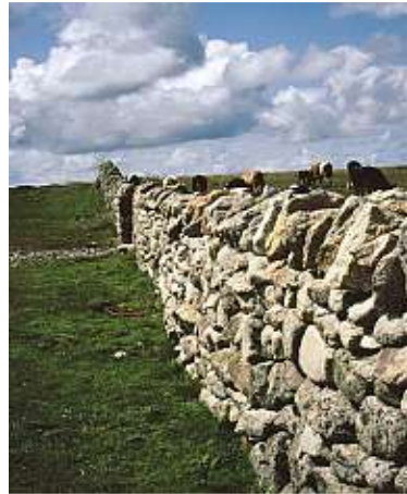
Rocks of Lundy Granite used to construct stone walls on the island
