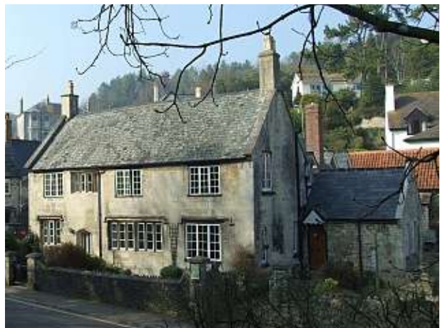
An important local house constructed of Beer Stone. Walls in ashlar stone with carved window lintels and door frames. Beer. ©DW Allen
